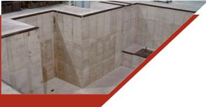
The project required excavation of a 24-foot deep pit. Crane columns located near the excavation had to be supported during construction to avoid any shifting or weakening of their base. By the end of July, the press had been set into place and NO adjustments were required.
